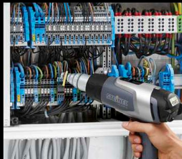
Shrinking cable sleeves in distribution cabinet
