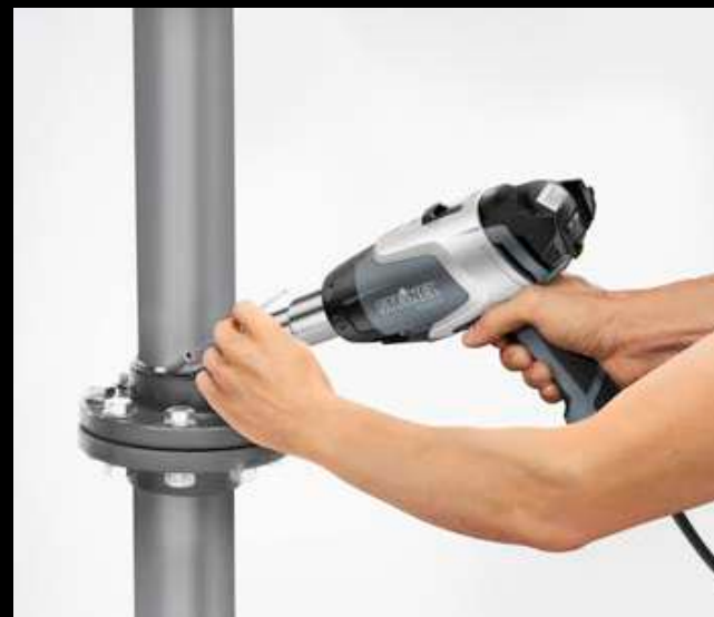
Welding plastic in tank and apparatus construction.
