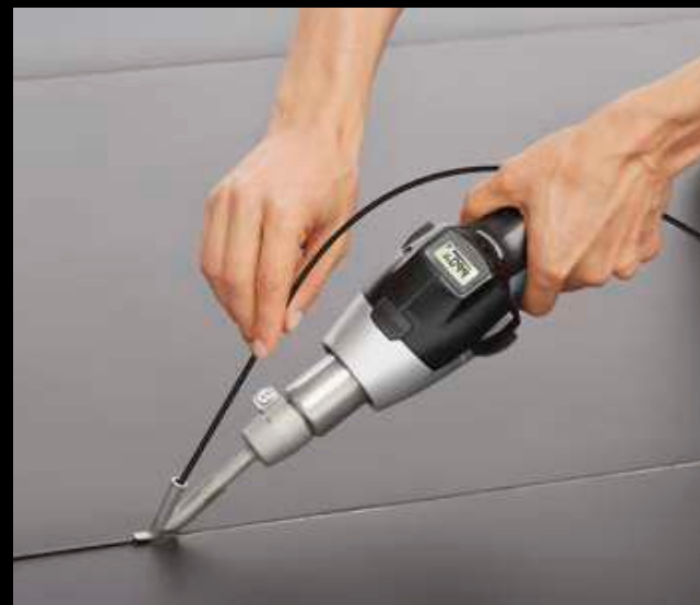
Welding linoleum floors.
