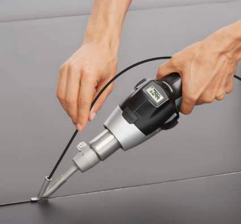
▲ Welding linoleum HG 2620 E
