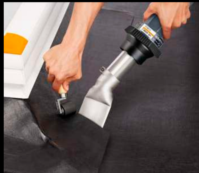
Overlap welding on a light dome.
